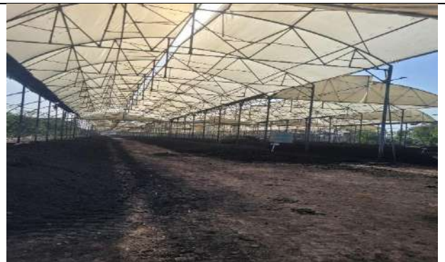
Photo 4: Covered compost yard at Ajeetpur site
