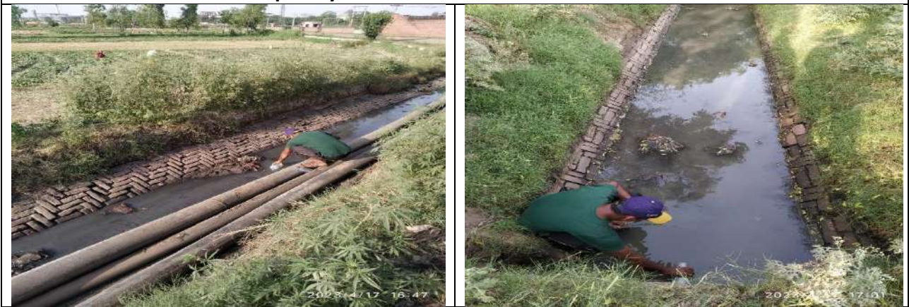
Photo 30: Drain u/s of Ajeetpur site bio-compost yard
