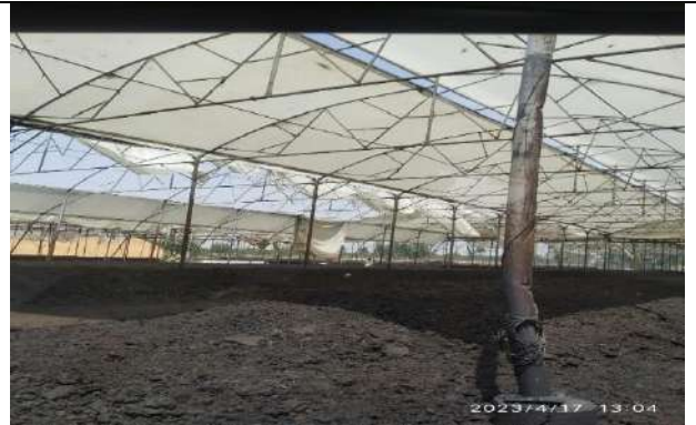
Photo 2: Covered compost yard at Hitachi site
