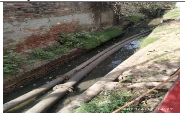
Photo 15: Drain near entrance gate of unit
