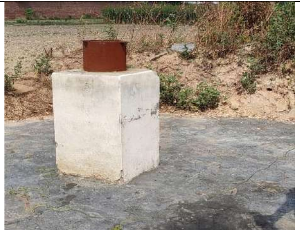
Pic.-14 Piezometer well no.- 06 at Ajeetpur Bio-compost Site (28.768208, 79.029999)
