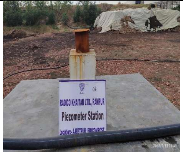
Pic.-12 Piezometer well no.- 04 at Ajeetpur Bio-compost Site (28.768670, 79.030653)
