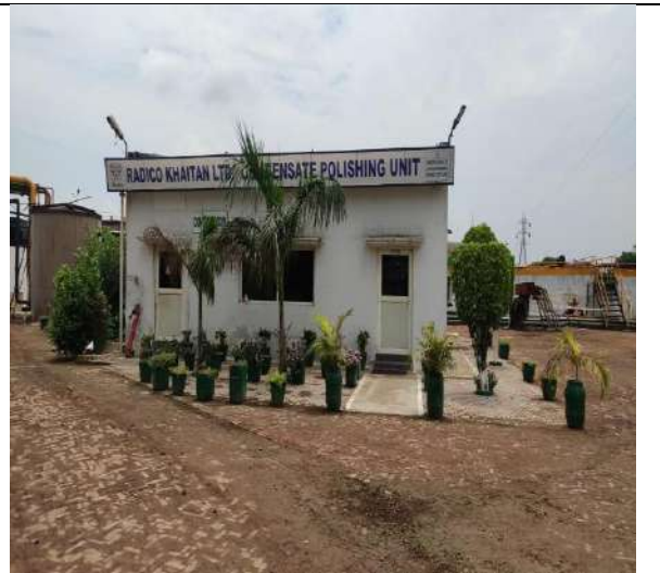
Pic.-21. CPU control room
